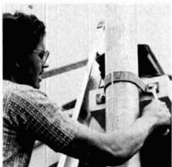
Mounting the House Bracket
